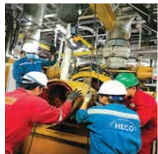
STATOR Checking - Cleaning - Drying - Varnish Insulation
