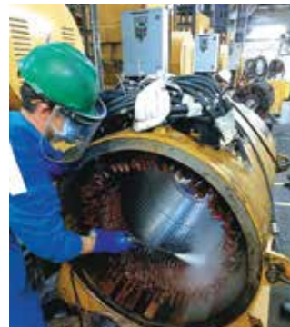
STATOR Checking - Cleaning - Drying - Varnish Insulation
